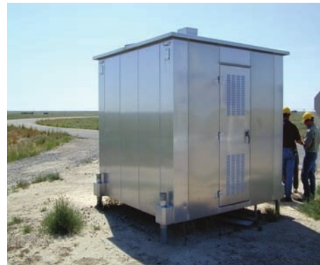
Figure 6-4. Grade Crossing Shelter and Sensor Connection
