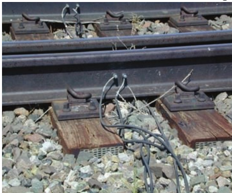
Figure 6-4. Grade Crossing Shelter and Sensor Connection
