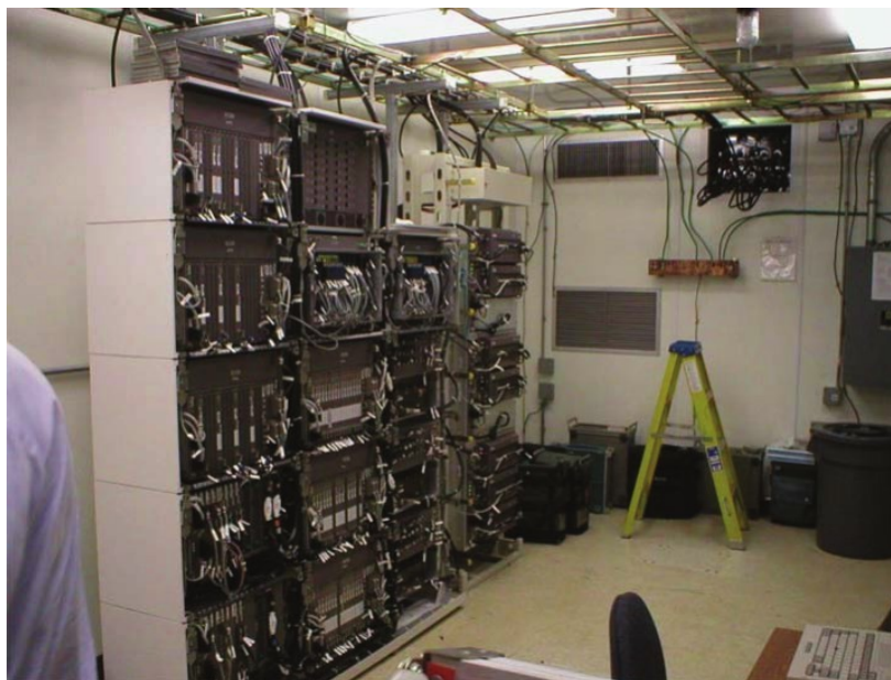
Figure 3-4. Cellular Base Station Equipment
