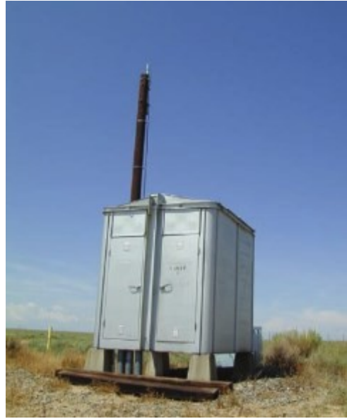
Figure 6-3. Typical Block Signal Control Equipment Enclosure
