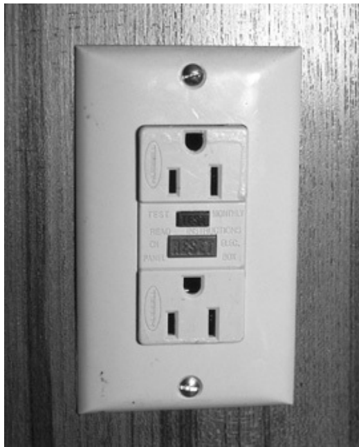
U.S.-style GFCI-protected outlet. To test, push the red button. To reset, push the black.
