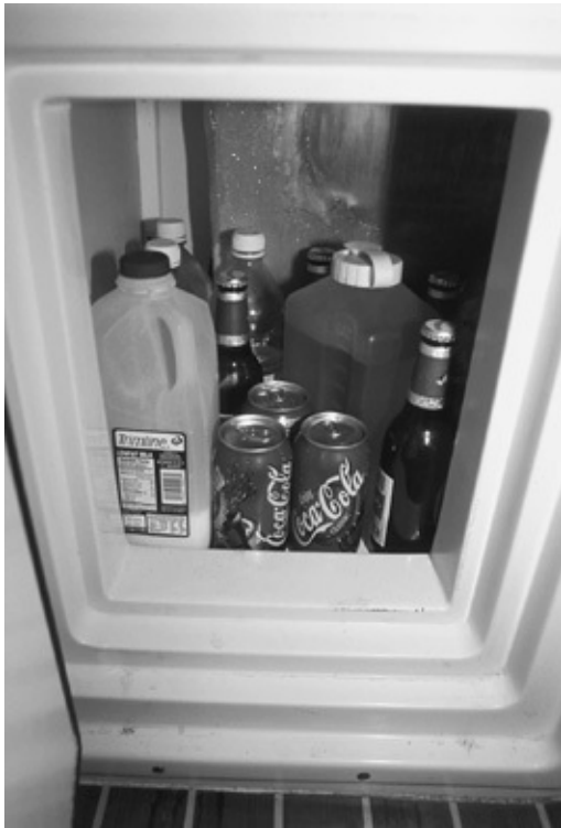
A well-constructed and sealed small front-opening door at the base of the refrigerator icebox greatly improves access.
