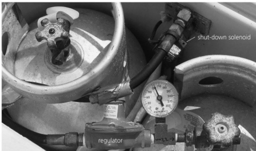
Detail of the previous installation. It's a bit of a tight fit, with potential chafe points on the gas hose that have been protected with duct tape. The remotely controlled shut-down solenoid is on the low-pressure side of the regulator. These are old-style U.S. gas bottles.
