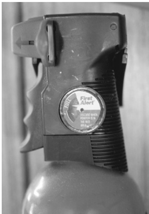
Pressure gauge on a fire extinguisher. These need to be regularly checked. Dry-powder extinguishers also should be inverted periodically to keep the powder from caking up.
