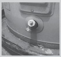
Drain valve on water heater (requires flat-head screwdriver)
