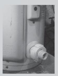
Drain valve with hand-turn knob
